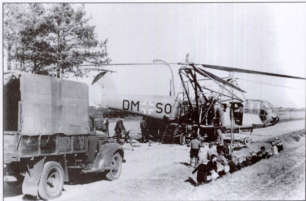
Fa 223 Drache V11 DM+SO, damaged during rescue operation in Holland in May 1944, being overhauled in the field.
