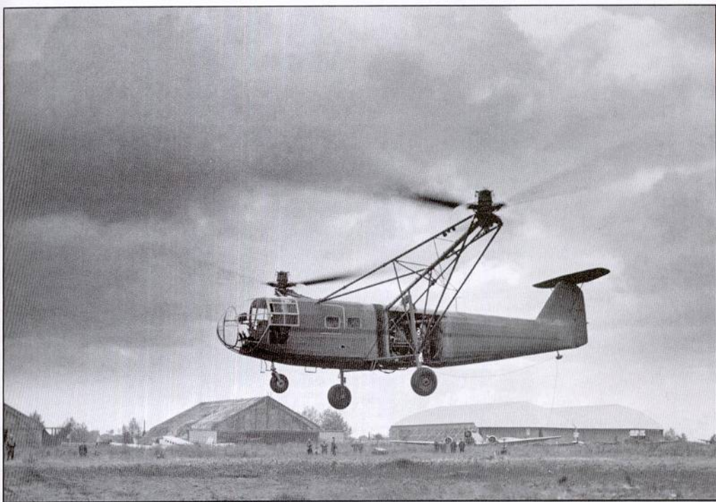
SE 3000, the French version of the Fa 223, Drache during factory tests (1948)
